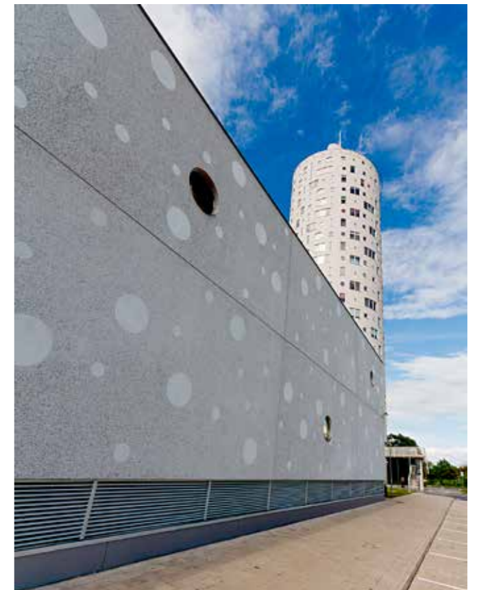
Ahhaa teaduskeskuse pesubetonist välissein, taamal Tigutorn, 2009. The outer wall of the Ahhaa Science Centre is made of exposed aggregate concrete; in the distance is the Snail Tower, 2009.
